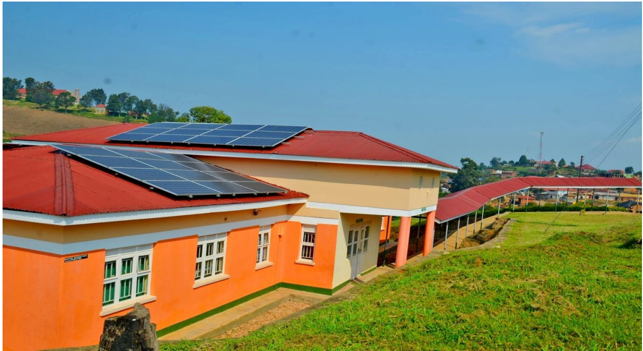
Kanungu HC IV, Kataate Hospital Project Operation Theatre built by the generosity of Germans led by Dr. Holger Listle.
